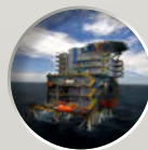
OFFSHORE PLATFORMS AND SERVICES
