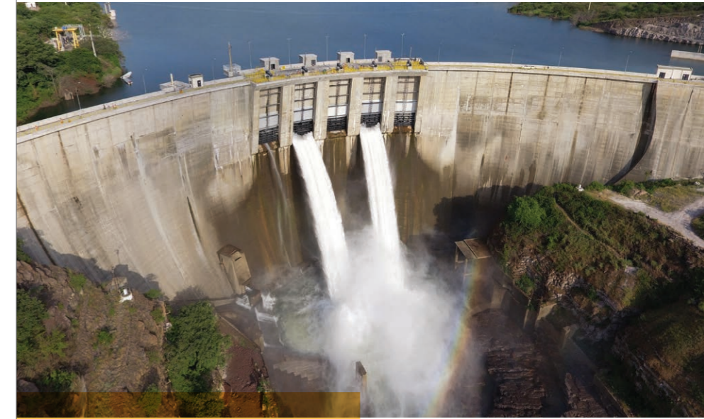
Laúca Hydroelectric Plant – Angola
