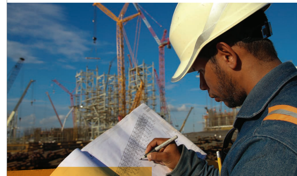
Punta Catalina Thermoelectric Plant – Dominican Republic
