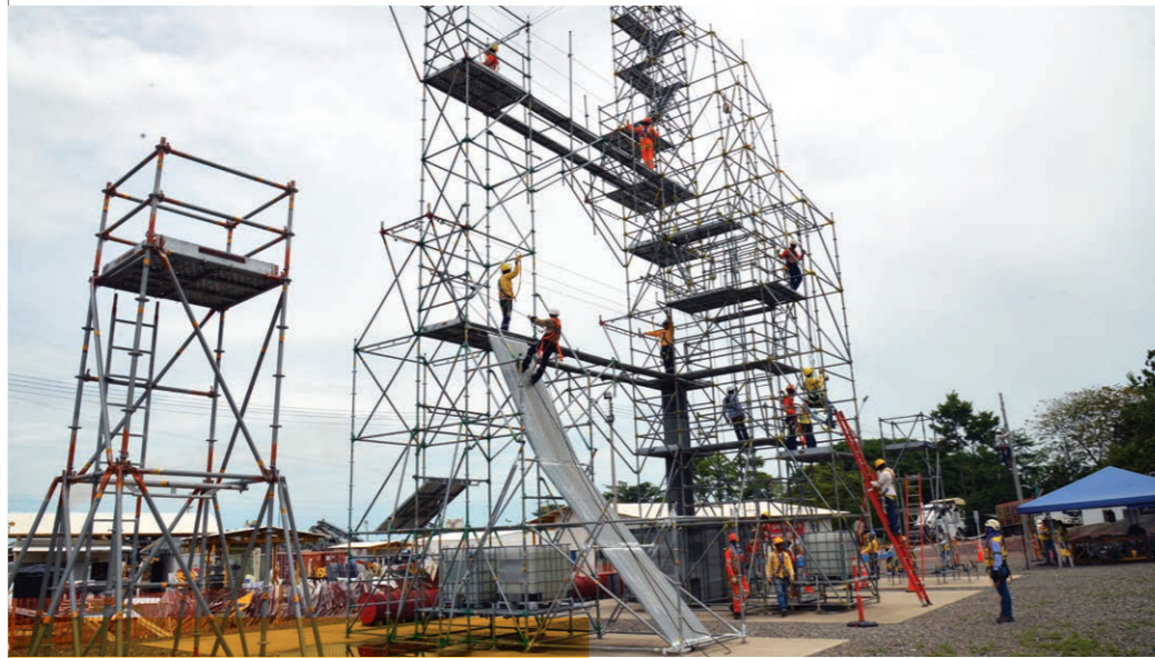
Training Camp for Working at Heights - Colombia
