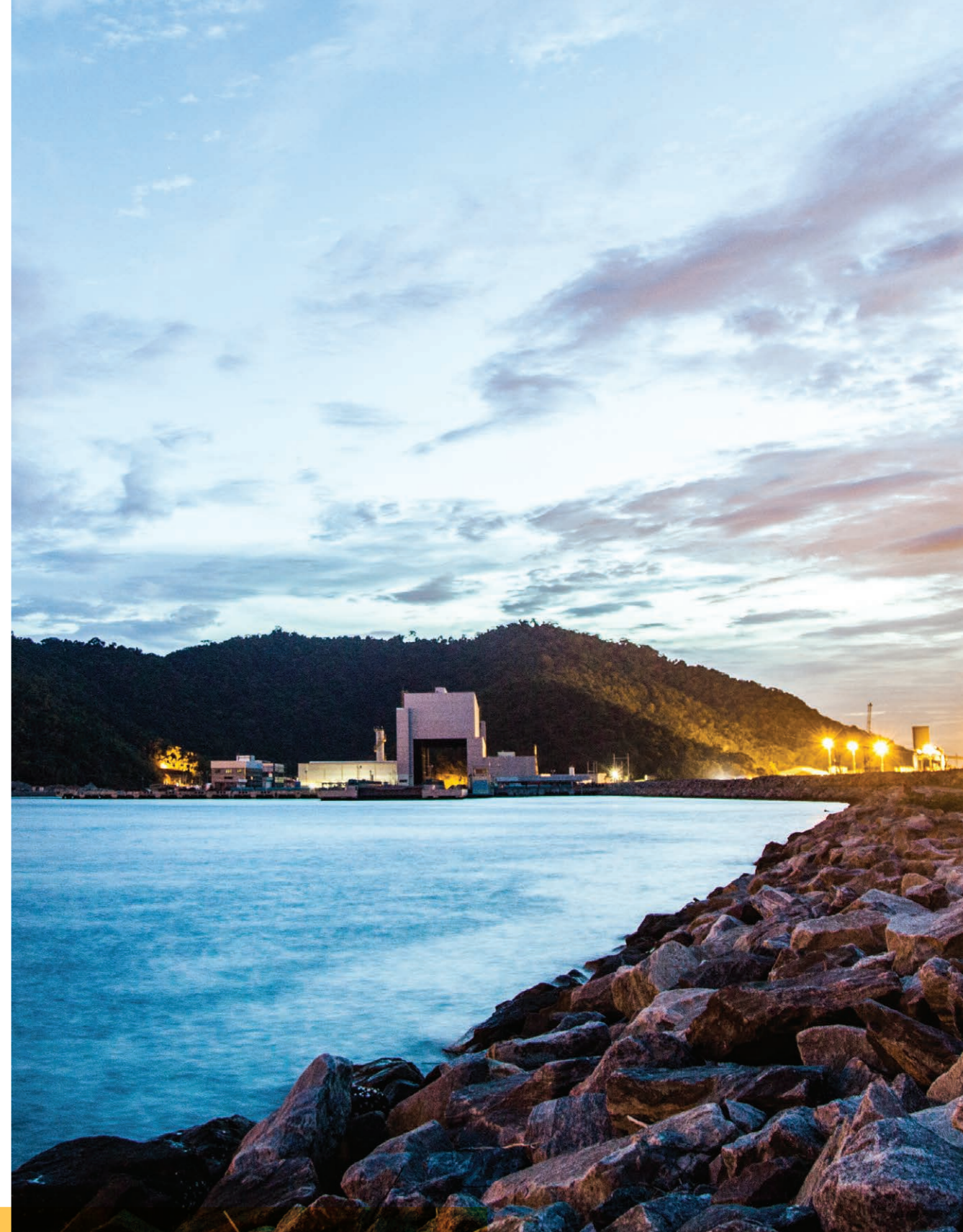
Shipyards Project, Rio de Janeiro - Brazil
